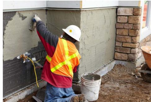
Moisture curing the mortar scratch coat may help reduce cracking and ensure proper hydration during curing. Before applying manufactured stone veneer, the mortar scratch coat can be dampened so that the surface appears wet but free of standing water. It is acceptable to install stone on a fresh mortar scratch coat once it has obtained a workable texture such as thumbprint hard.
