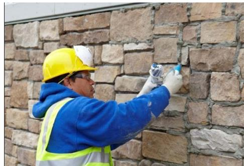
If the manufactured stone veneer is inadvertently moved after initial set has begun, it should be removed, mortar scraped off the back of the manufactured stone veneer and scratch coat, and then reinstalled following the application process. Install manufactured stone veneer from the top down when possible to minimize cleanup requirements.
