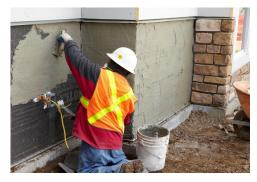
and ensure proper hydration during curing. Before applying manufactured stone veneer, the mortar scratch coat can be dampened so that the surface appears wet but free of standing water. It is acceptable to install stone on a fresh mortar scratch coat once it has obtained a workable texture such as thumbprint hard.
