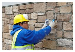
few seconds of the setting movement process. At this point, no further movement of that manufactured stone veneer should be made as bonding will be broken.
